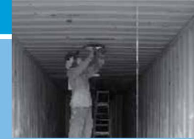
Cut out the opening for the turbine ventilator and weld a (4") inch circular turbine base to the opening. (The base must not stick out more than (2") inches).
