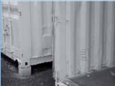
Apply 2 coats of anti-corrosion white paint inside and outside the container. Cover the air vents on the inside with mosquito screening to prevent insect infestation.
