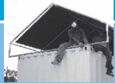
Build a roof (canopy structure, tin roofing, ...) preferable with an angle of 120° and fix it to the container.
