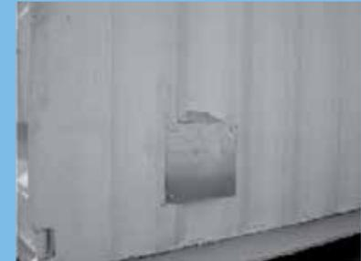
Cover these air vents on the outside with home made moulded galvanized steel plates welded 3/4 around to prevent vertical & lateral water infiltration.
