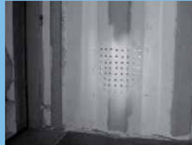
Make 4 to 8 rodent proof lower lateral 12" x 12" air vents by drilling series of 1/2" holes through the inner groove of the container wall. (Inside view)
