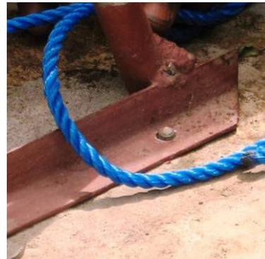
3) If the bolt is too short to fix the nut, use a hammer and a chisel (or at least a screwdriver flat) to brake thin layers of the cement by mortising slowly the surface around the bolt
