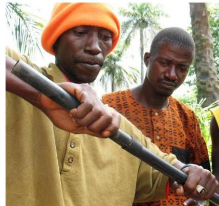
**Do not remove the small pipe while the flare is still hot**
