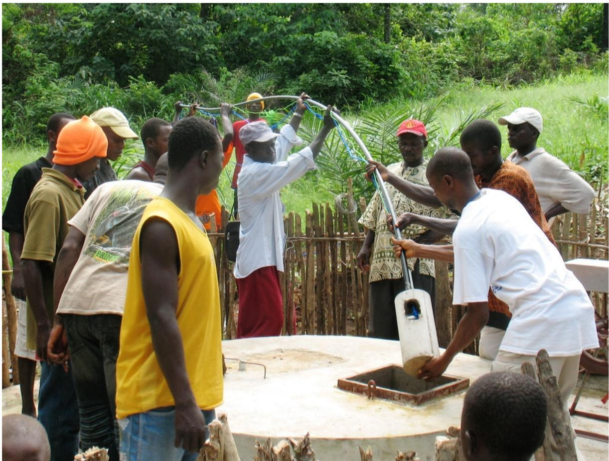
**Don't turn the pipe around during installation to prevent the rope from winding around the pipe. Lower it straight. Keep the rope on one side of the pipe.**
