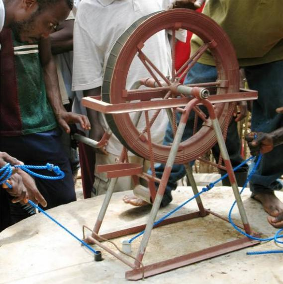
1) Place the wheel basement on the cover above the holes. Remove the pump cover
